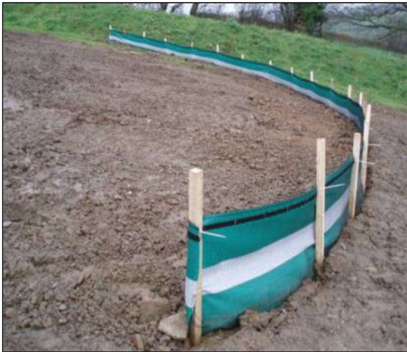
Plate 6.1: Fabric Silt Fencing at the toe of a slope
